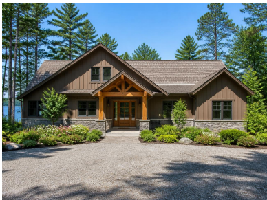
Front of Cottage
